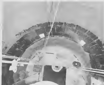
Looking down, inside process stack. Mirando abao, den process schoorsteen.
